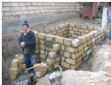
The Water Tank
